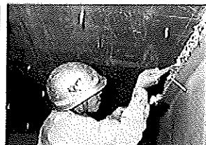
Sealing the plate periphery
